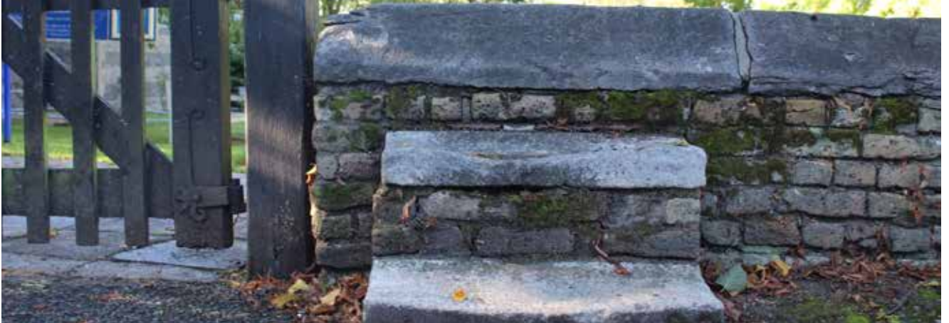
Figure 34: Boundary wall of the Church of St Mary
