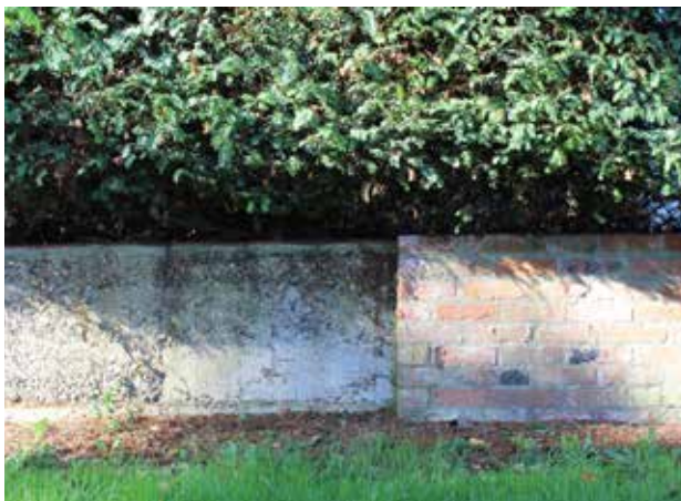
Figure 82: Replacement of low brick wall with concrete, which is out of keeping with the material palette of the area
