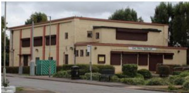
Figure 24 & 25: Bata Cinema © Bata & East Tilbury Village Hall
