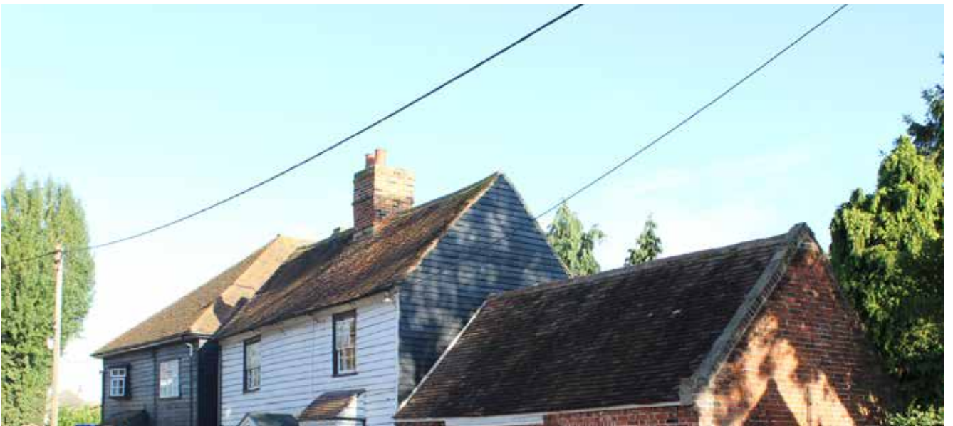
Figure 58-60 (clockwise from top left): Examples of roofing
