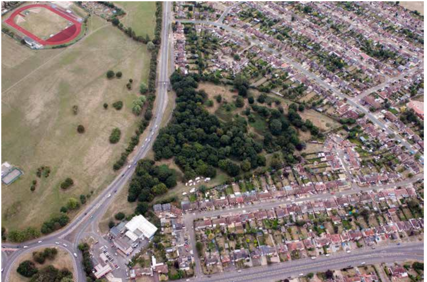
Figure 13 Hangman's Wood in its immediate setting. Some of the darker vegetation in the mown grass may indicate other dene hole sites.
