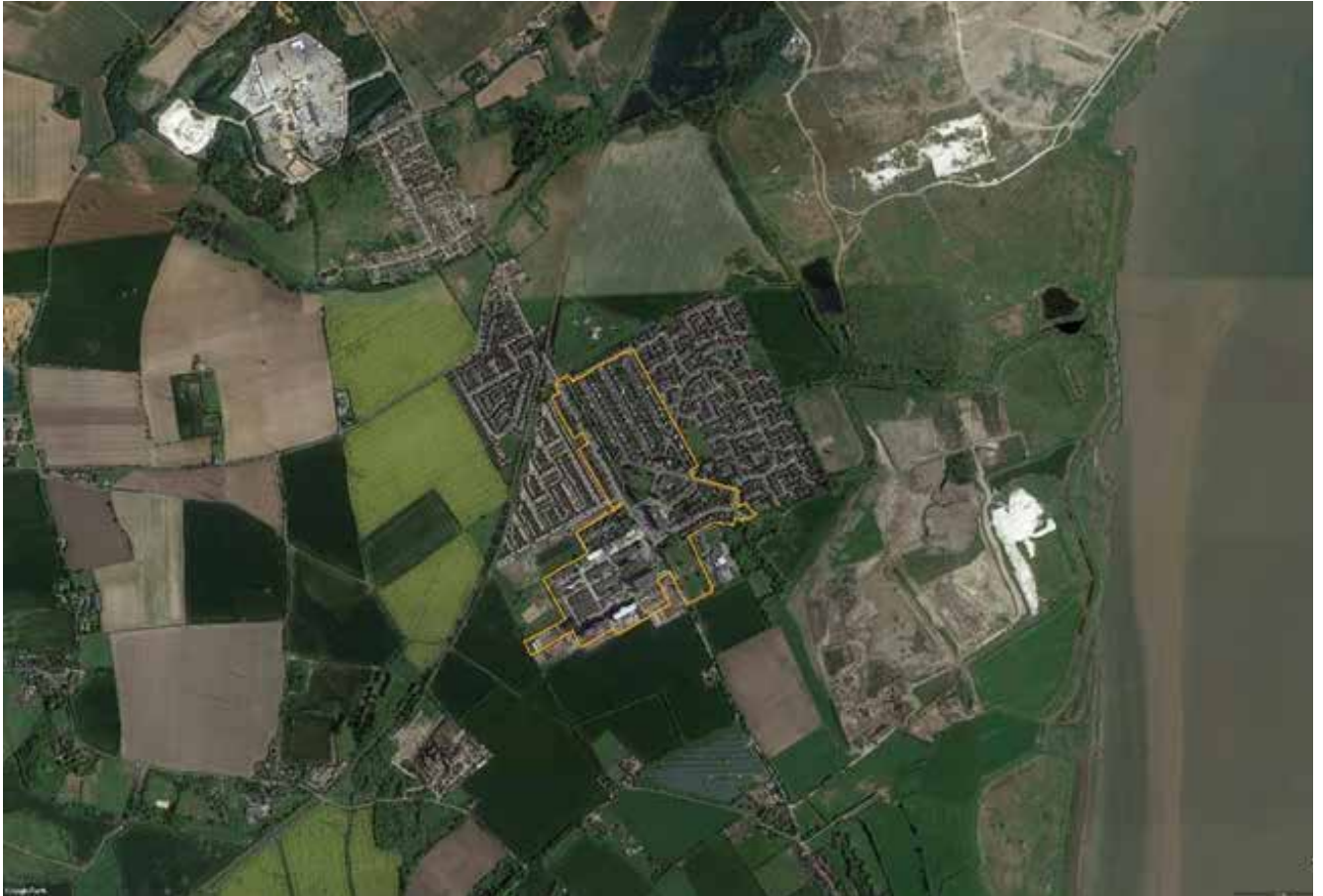
Figure 2: East Tilbury (Bata Village) Conservation Area within its wider context © Google Earth
