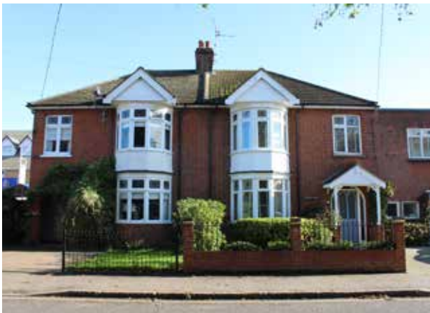
Figure 86: Two dwellings showing the impact of alterations. Window replacements, concrete roof tiles, porch and a garage extension have affected character.
